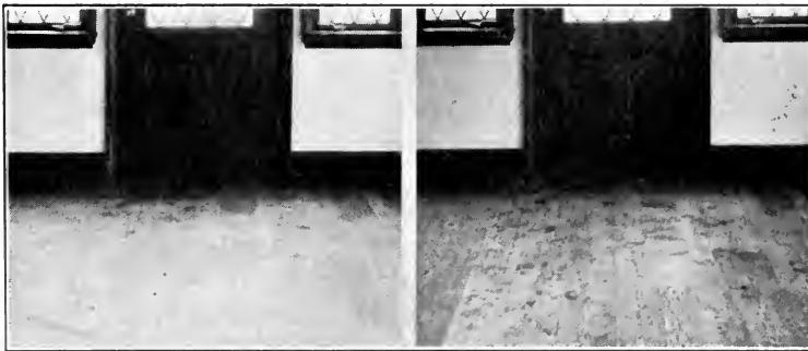
FIG. 6. Oak floor photographed with and without the Pola-screen over the lens, to subdue oblique glare in order to show grain and construction details.
